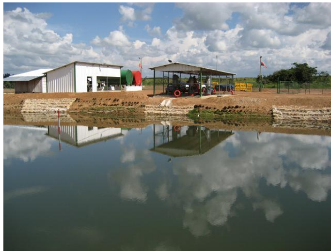
WACU CUNGO Project, Angola
